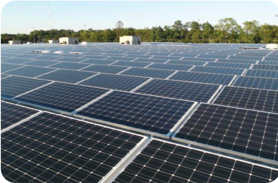
*In order to maximize available sunlight and space, the solar panels at OPEX are situated in six different directions, at various tilts.*
