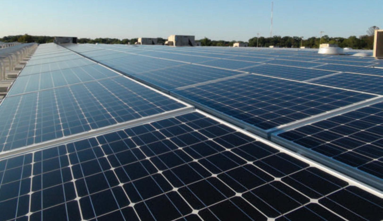
The factory and grounds now host 8,372 SunPower modules, with peak capacity of 2.77 megawatts.
