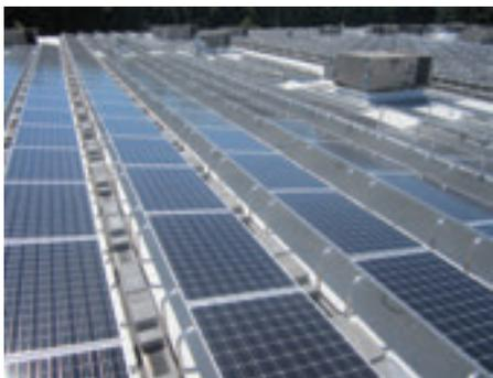
Modules are oriented in a variety of directions to optimize roof space and solar gain.
